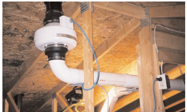
Sealing openings in the Foundation, and venting air up and out of the house can help reduce radon levels to acceptable levels.
